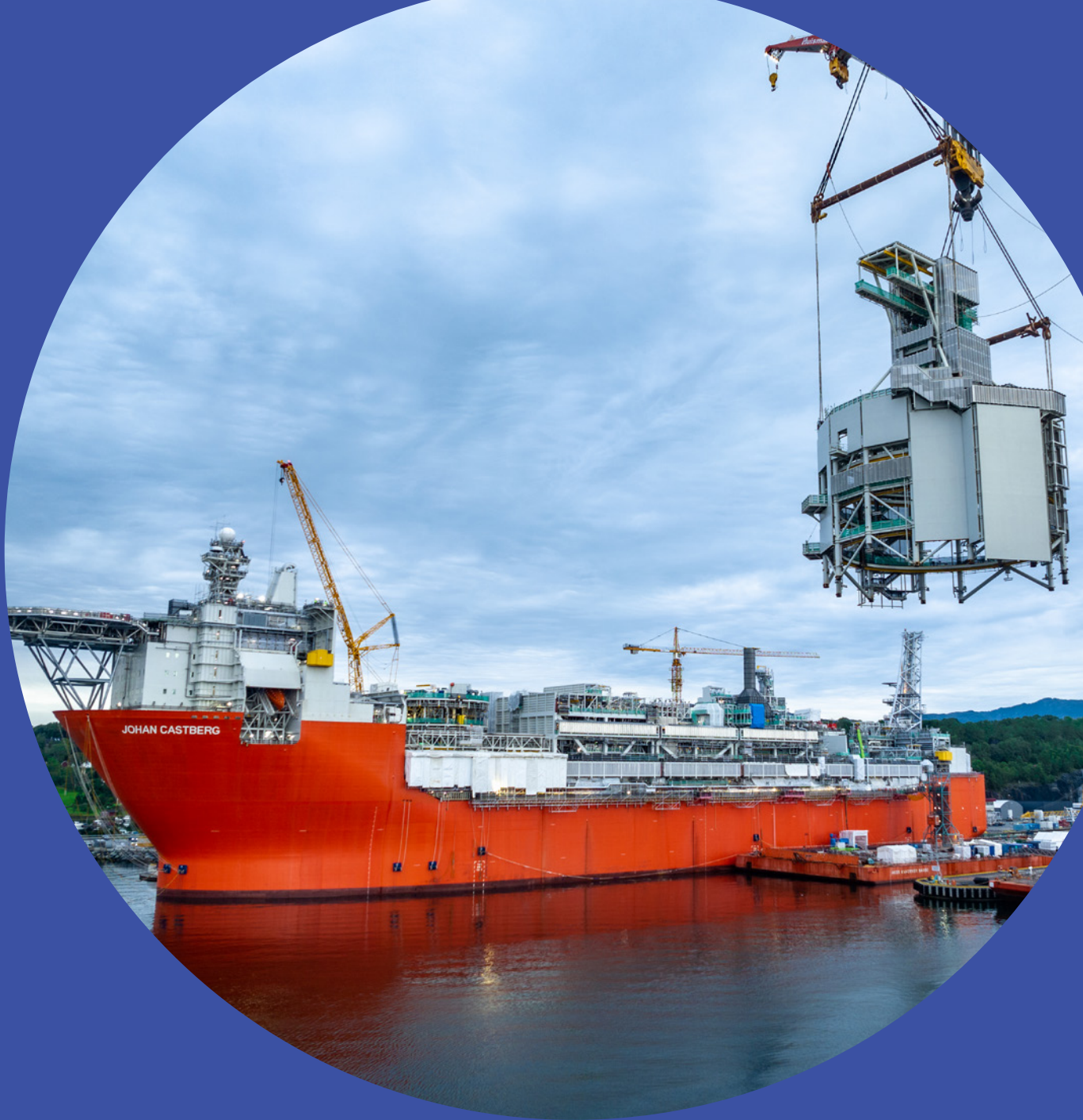
Final heavy lift completing Johan Castberg FPSO. Foto: Øyvind Gravås / ©Equinor
