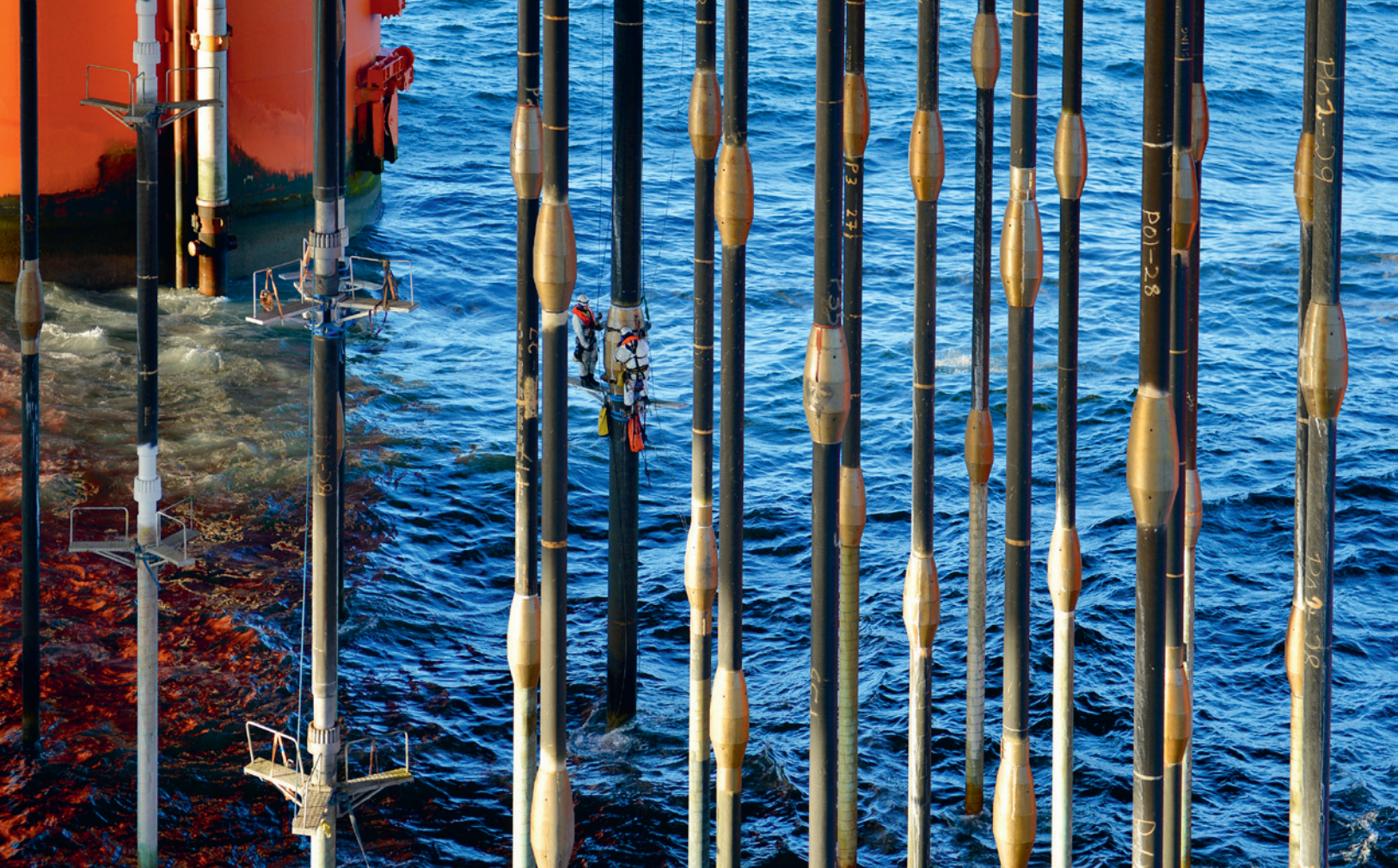
Risers on Snorre A. (Photo: Harald Pettersen/Statoil)
