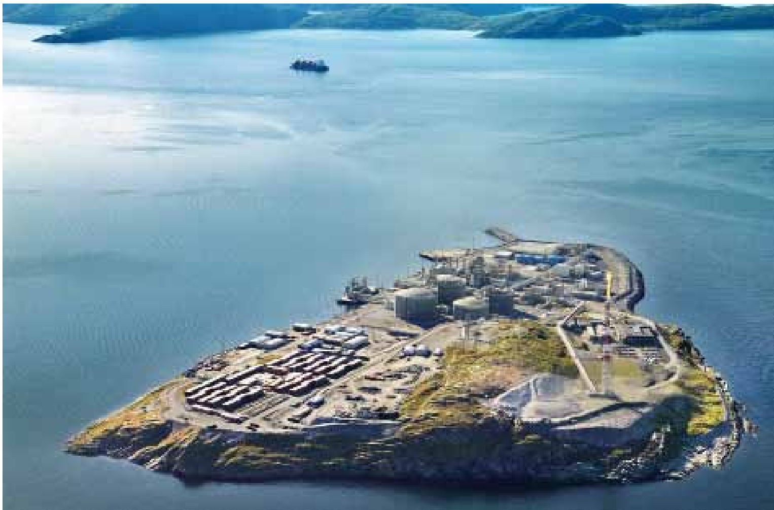
The Snøhvit gas liquefaction plant is the world's most northerly of its kind, and delivers energy to customers worldwide.
