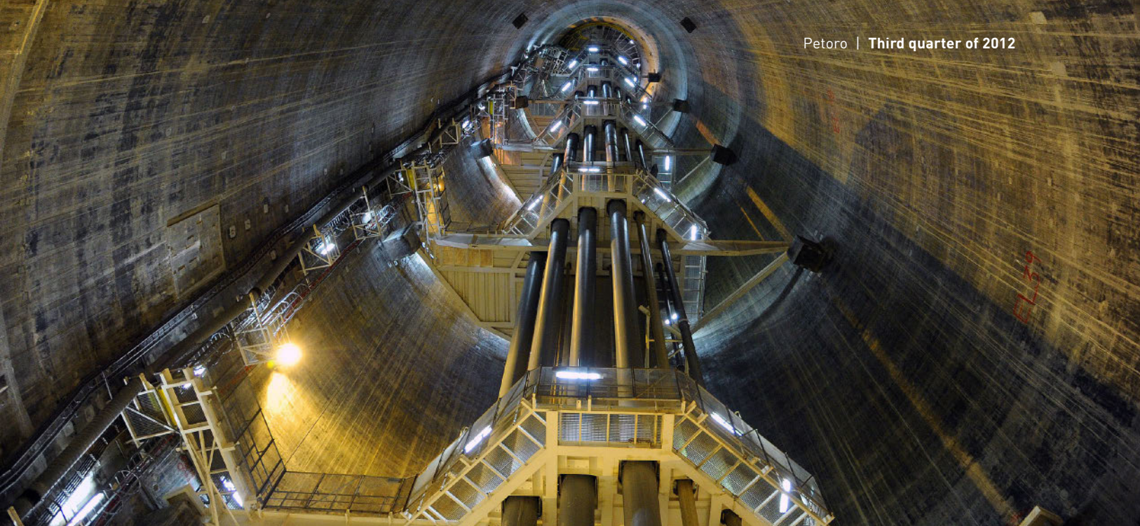
Support shaft on Troll A. (Photo: Harald Pettersen, Statoil)
