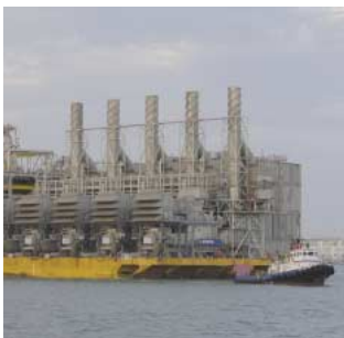
Preparing the Snøhvit process plant for shipment from Spain. Photo: Øyvind Hagen, Statoil.
