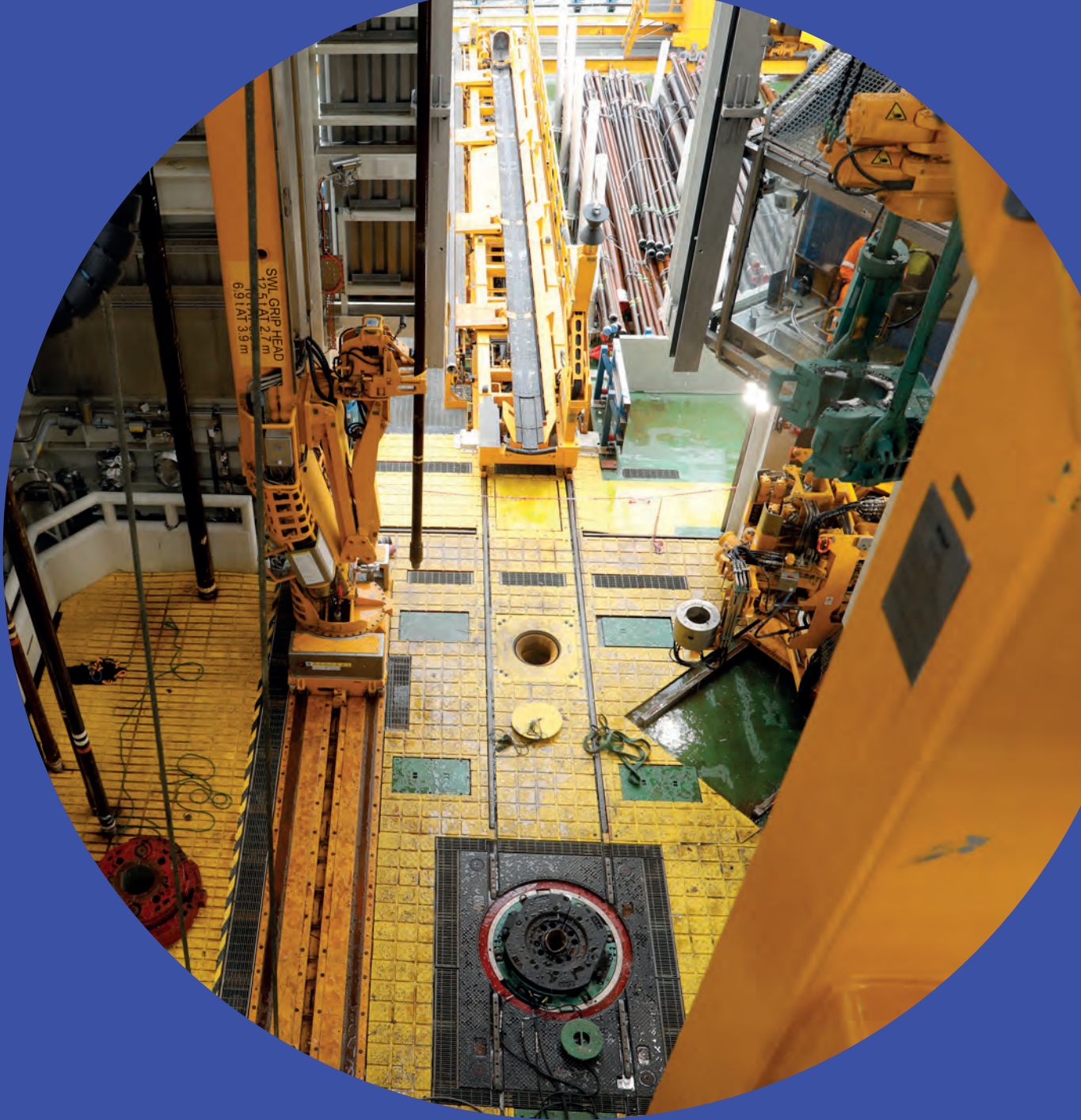
From the drilling floor at Johan Sverdrup. Photo: Arne Reidar Mortensen / Equinor
